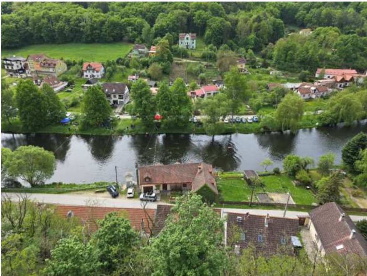
Fig. 3 River reach with installed cable ways
